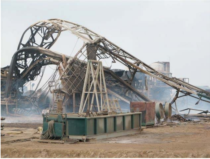
Figure 3: Wellbore blowout [Hamburger, (1983)]
